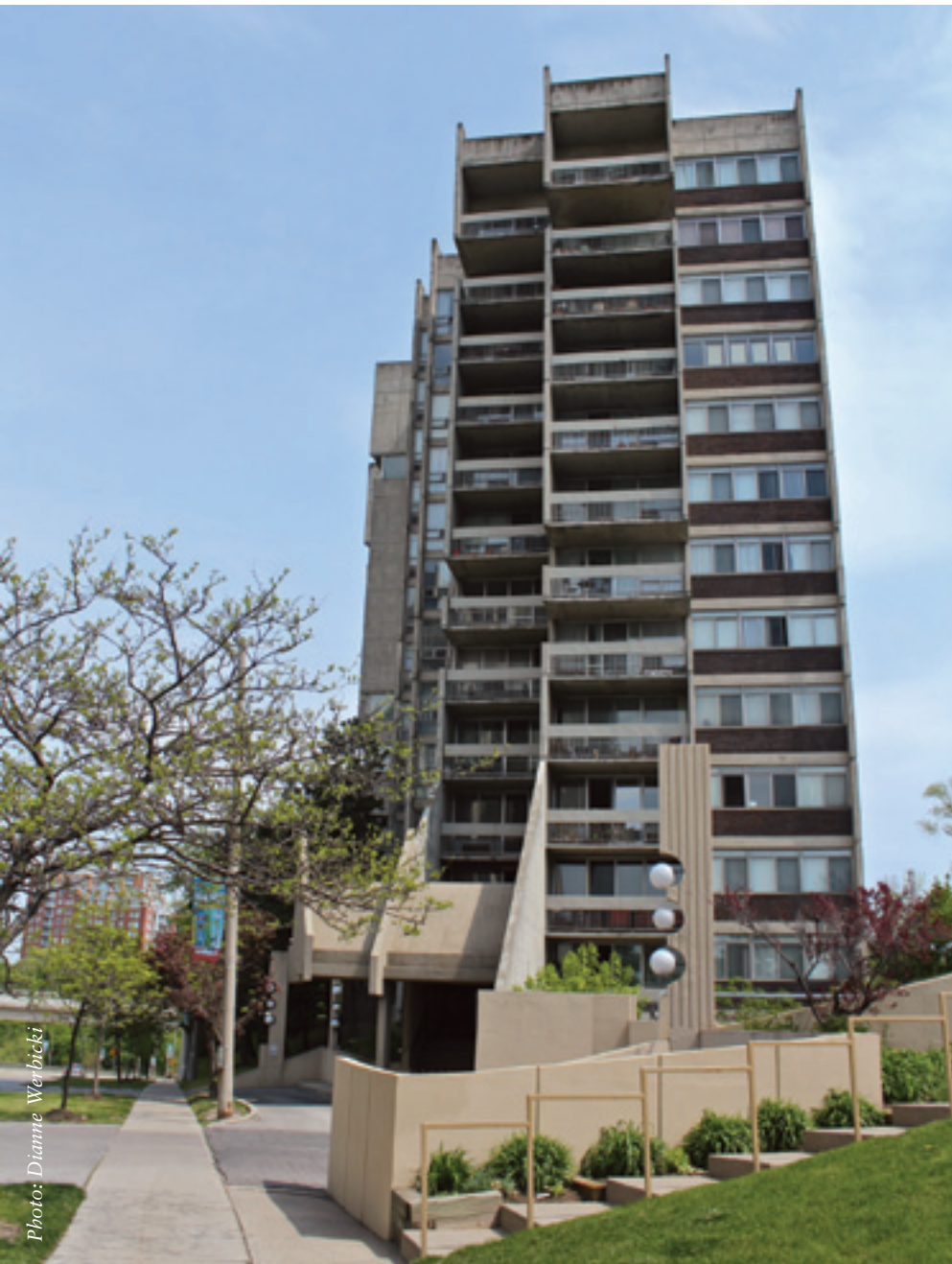
Oak Hill condominium on Speers Road in Oakville, Ontario was built in 1974.
