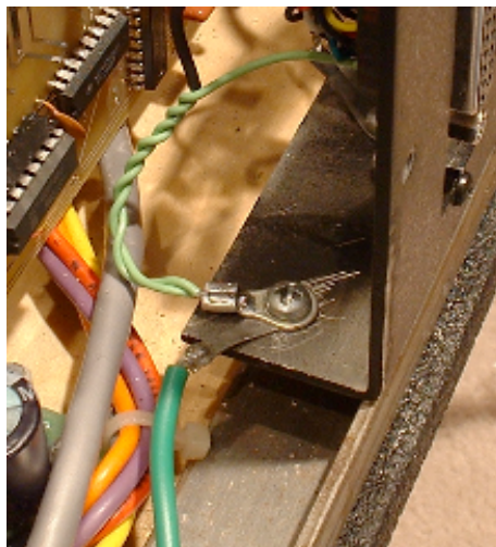
Figure 15: Cable Ground Connected to Panel Ground
