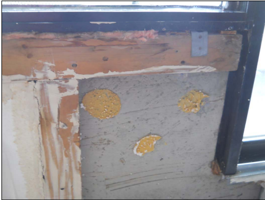
Photograph No. 23: 2" x 4" wood stud below fixed window frame
