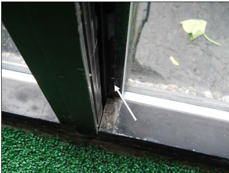
Photograph No. 14: Daylight visible through frame-to-glass junction - Pool
