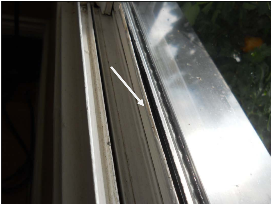
Photograph No. 10: Bedroom window frame bowed inward - Suite 1201
