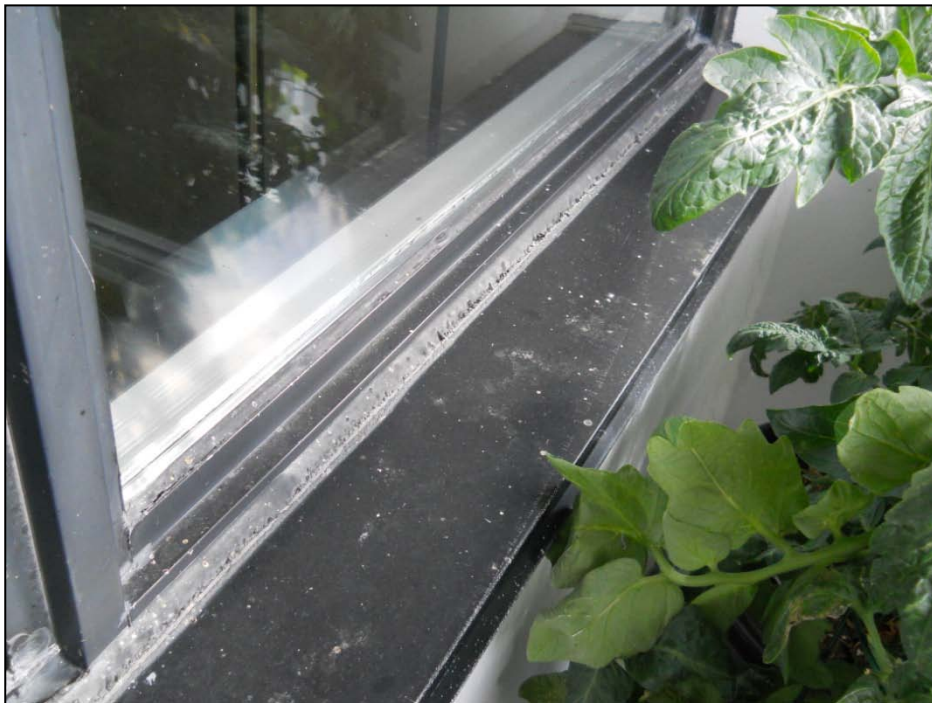
Photograph No. 12: Aluminum flashing added where there was a cracked concrete sill – Suite 1201
