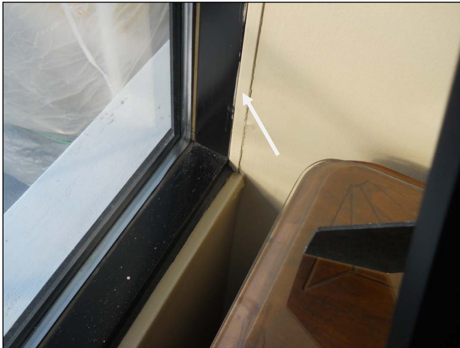
Photograph No. 18: Gypsum metal track fastened into window frame stop
