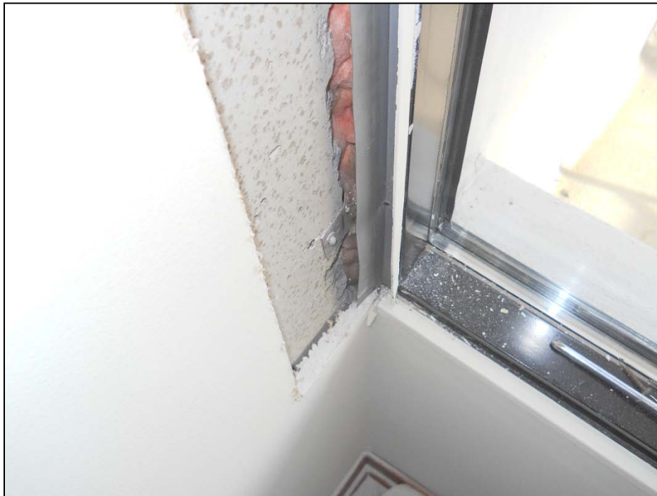
Photograph No. 25: Concrete chipped out to accommodate for window frame
