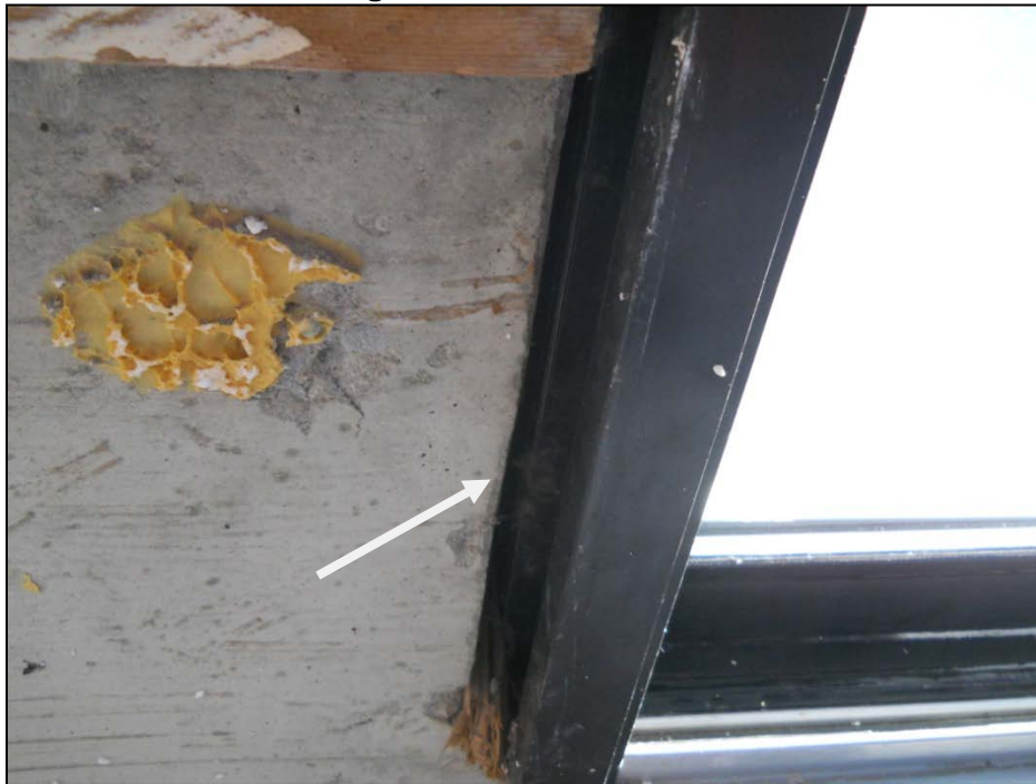
Photograph No. 22: No insulation present between sliding door frame & concrete
