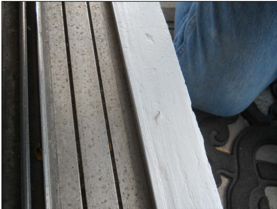
Photograph No. 16: Balcony sliding door frame sits directly on concrete curb
