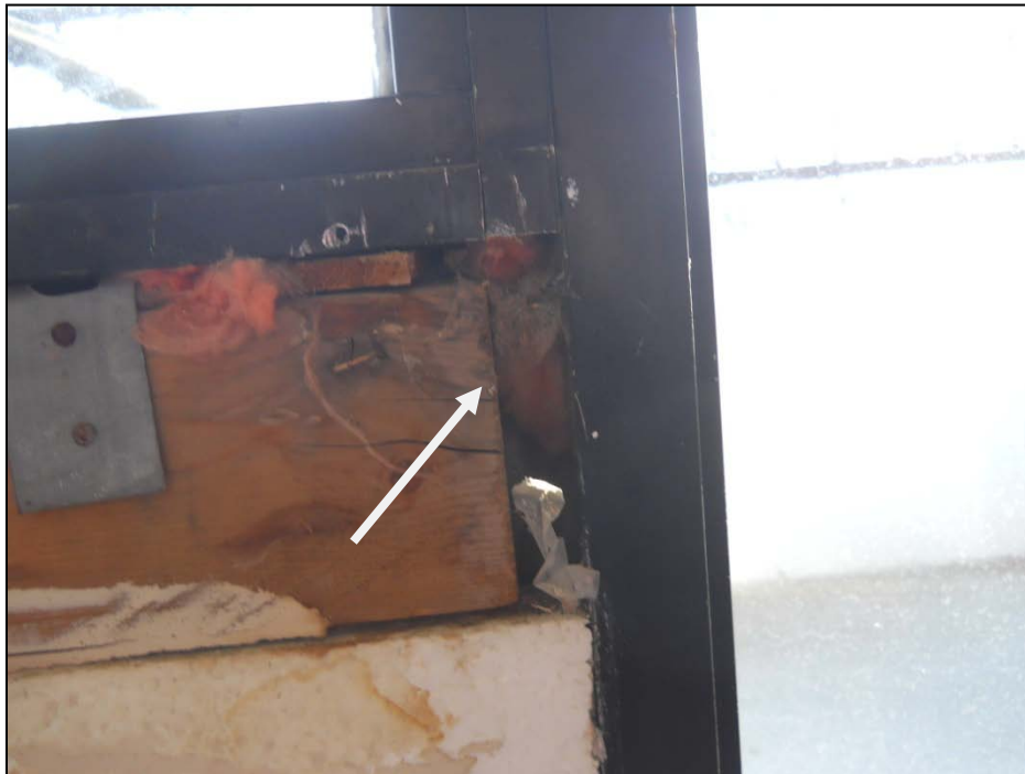
Photograph No. 24: Fibreglass insulation pushed between window frame & exterior concrete
