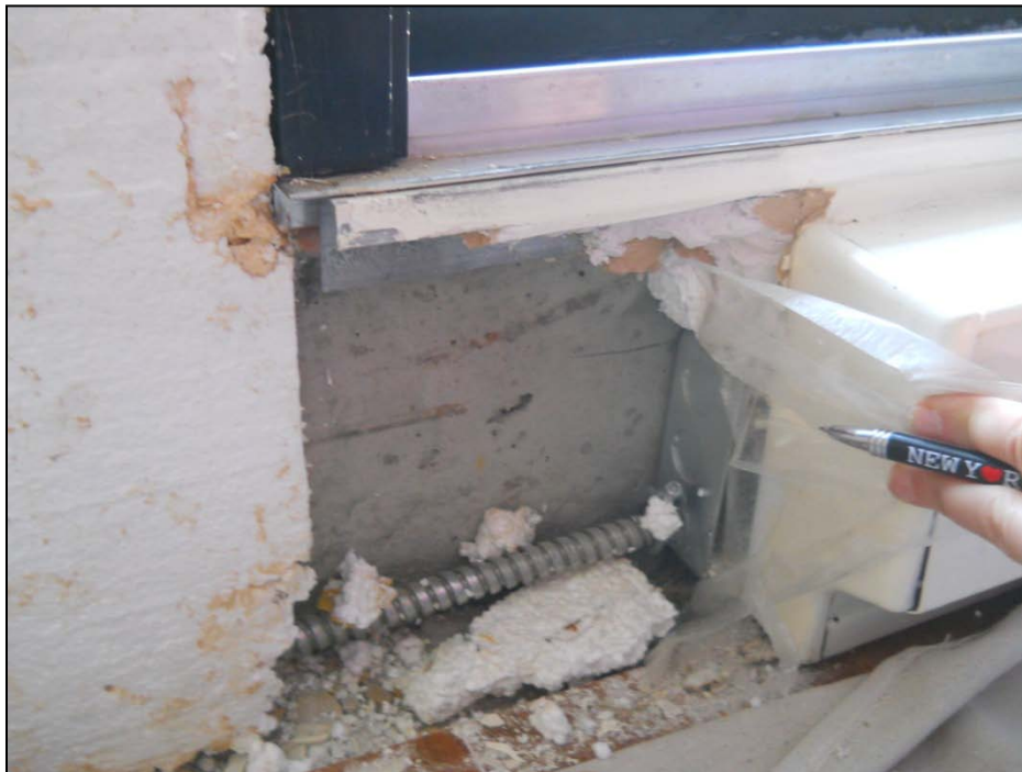
Photograph No. 20: Exposed 6½" concrete & electrical conduit
