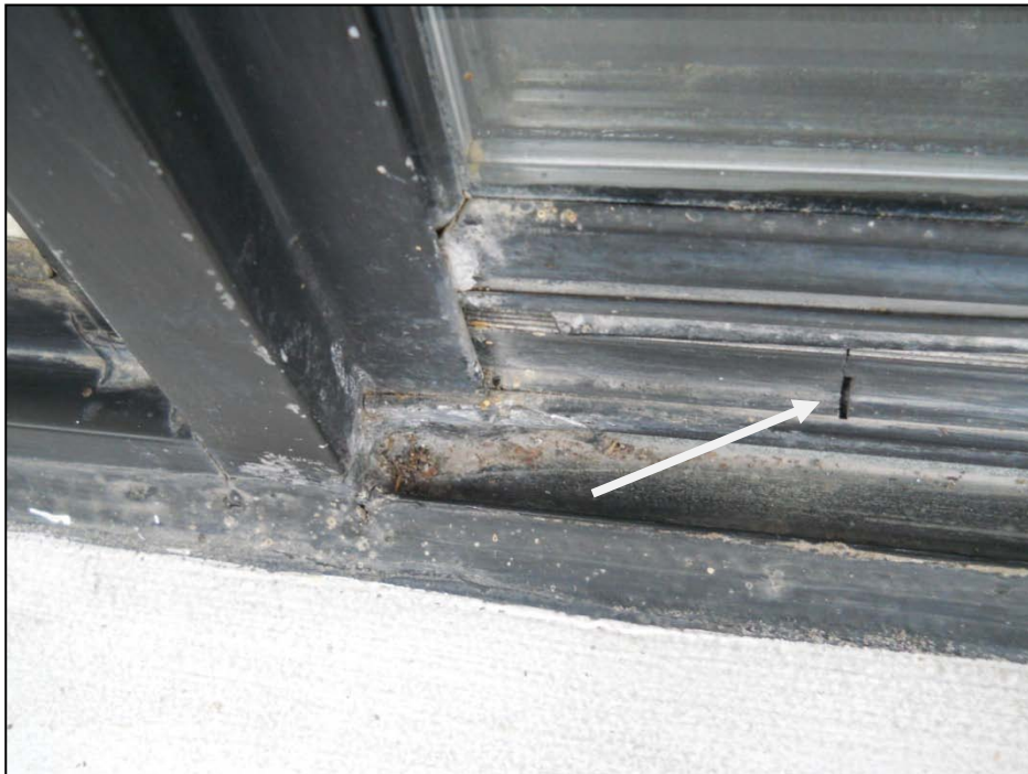
Photograph No. 4: Crack in aluminum frame in operable section - Suite 407
