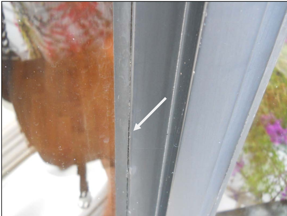
Photograph No. 8: Added heel bead sealant failing - Suite 1201
