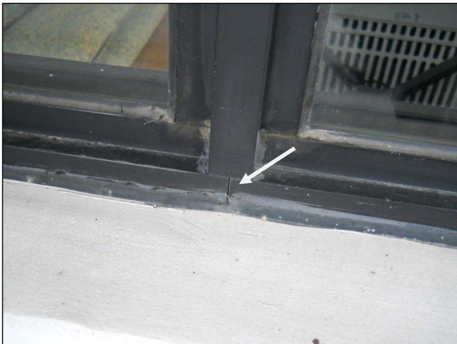
Photograph No. 2: Failed sealed joints within aluminum frame - Suite 407
