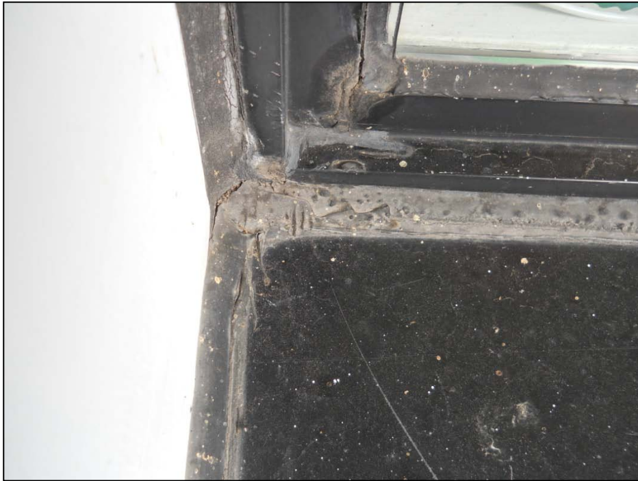
Photograph No. 11: Sealant at frame-to-wall connection brittle & cracked - Suite 1201
