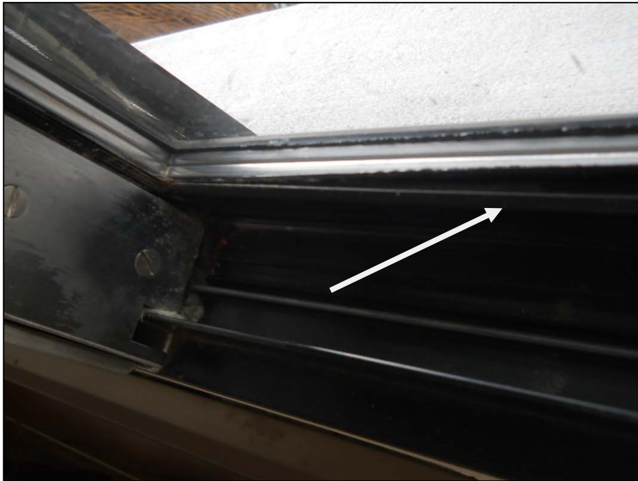
Photograph No. 5: Aluminum frame in bedroom bowed inward - Suite 407
