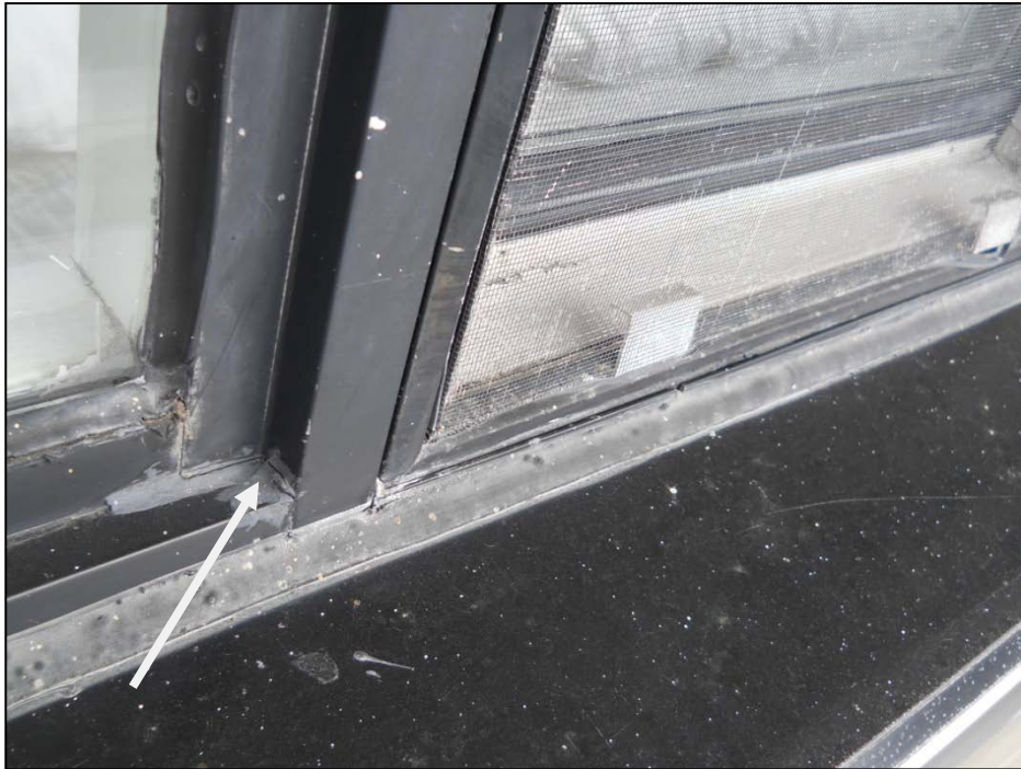
Photograph No. 9: Attempt to seal exterior joints in aluminum frame - Suite 1201
