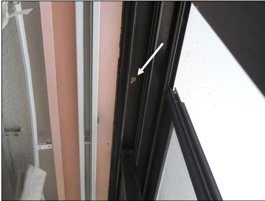
Photograph No. 15: Sliding door anchored into concrete slab
