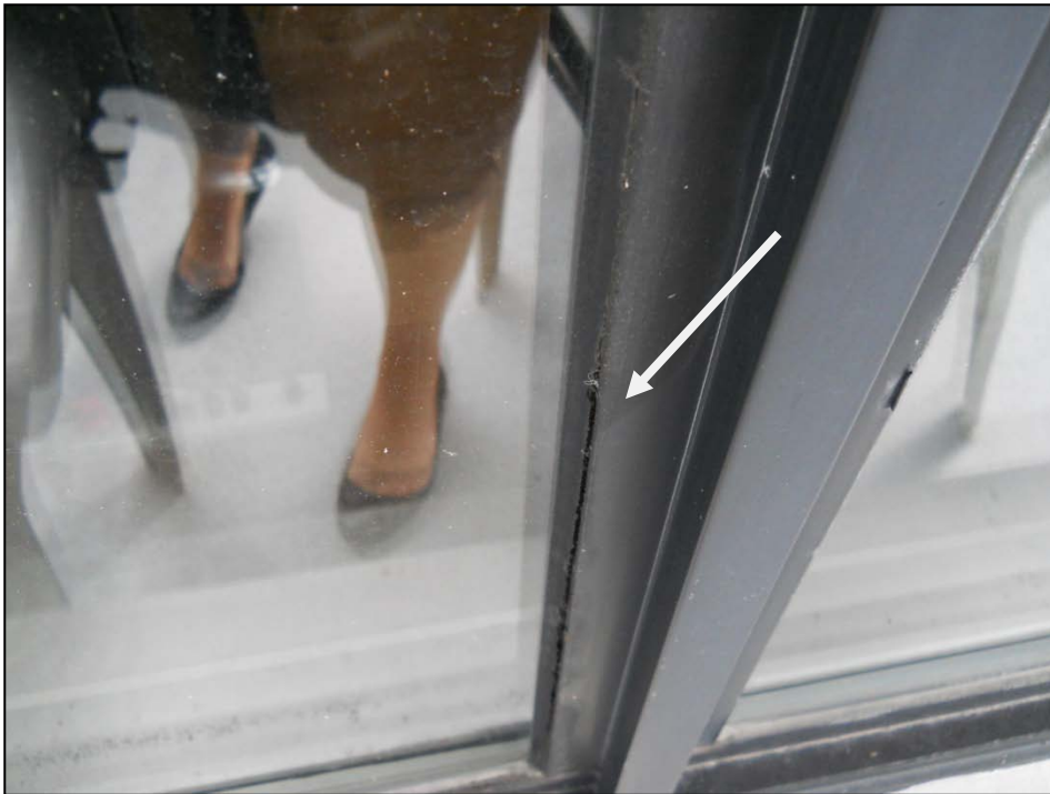
Photograph No. 1: Failed heel bead sealant at glazing-to-frame junction - Suite 407
