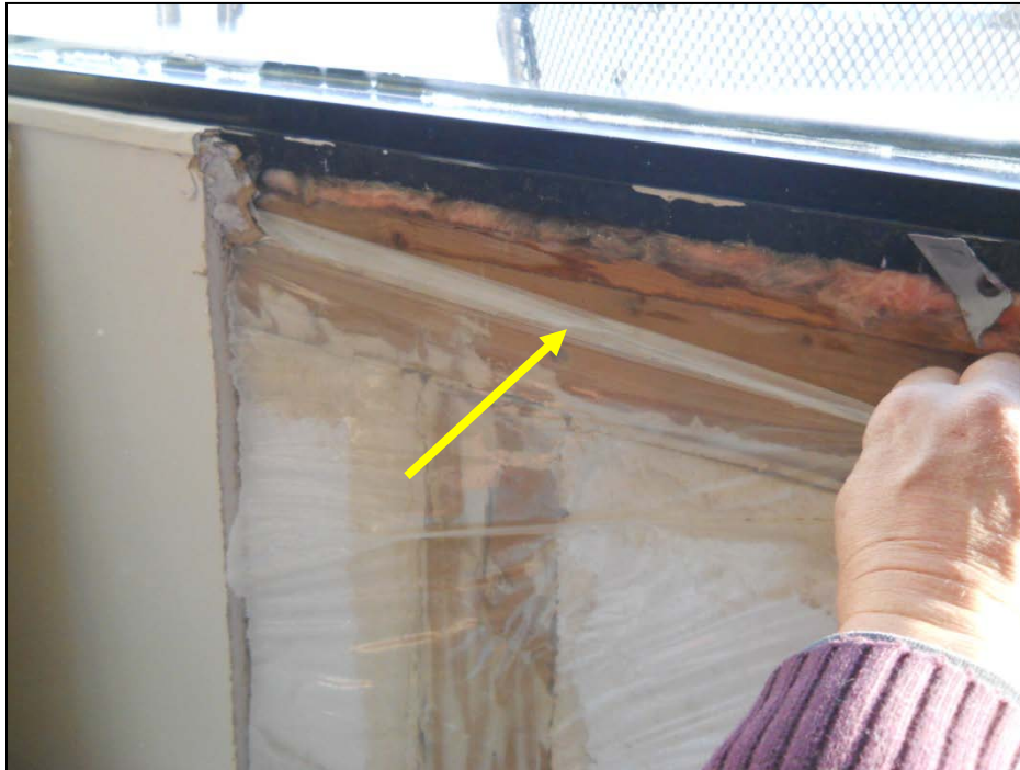
Photograph No. 19: Polyethylene Vapour Retarder (very thin)
