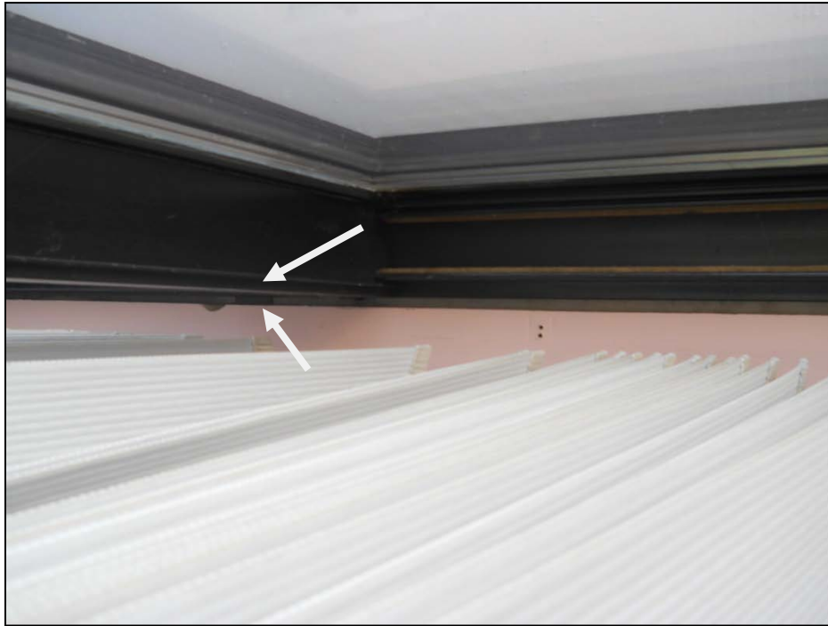
Photograph No. 17: Anchor clips fastening at fixed windows
