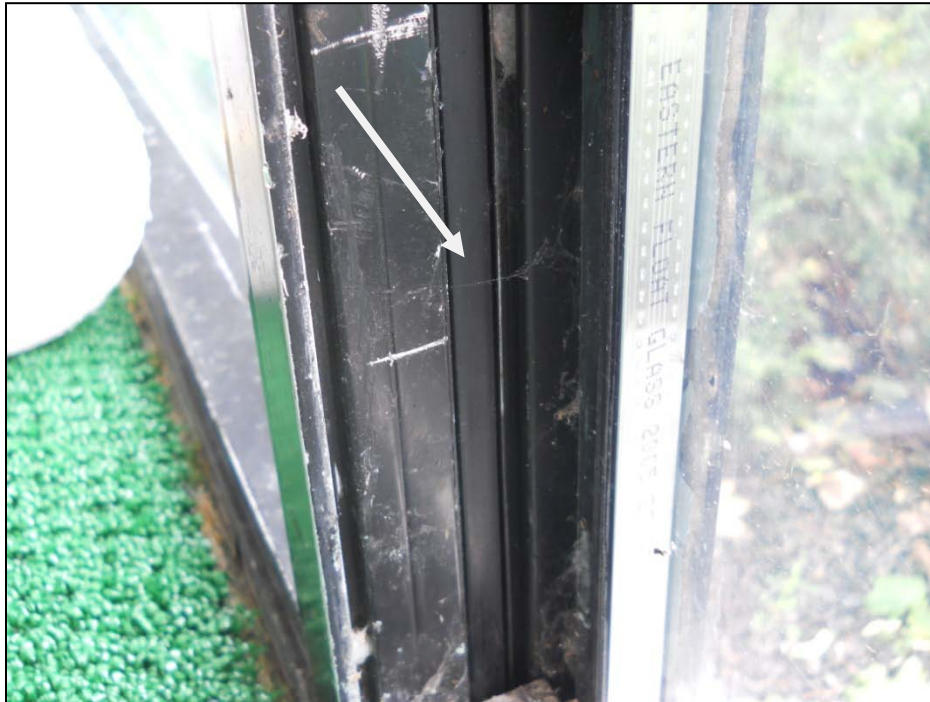
Photograph No. 13: Thermal break located at the interior of glazing
