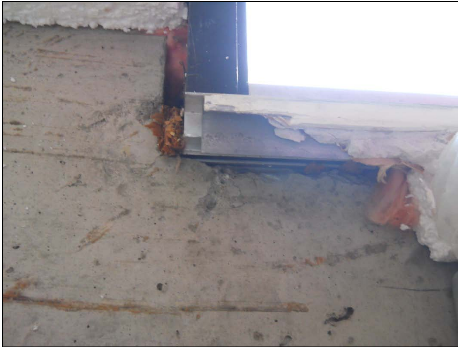
Photograph No. 21: Limited insulation present between sliding door sill & concrete curb
