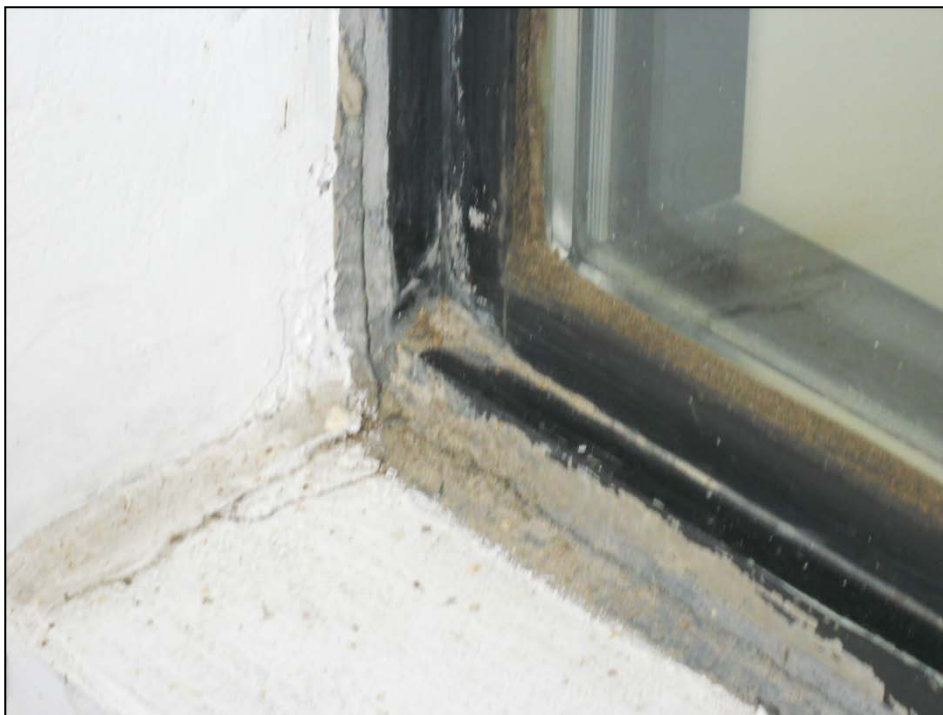
Photograph No. 6: Sealant at frame-to-wall connection brittle & cracked - Suite 407
