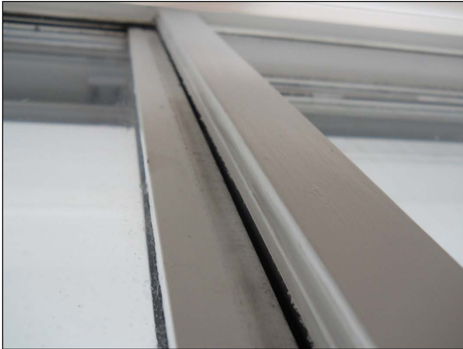
Photograph No. 7: Operable sliding door out of square – Suite 1201
