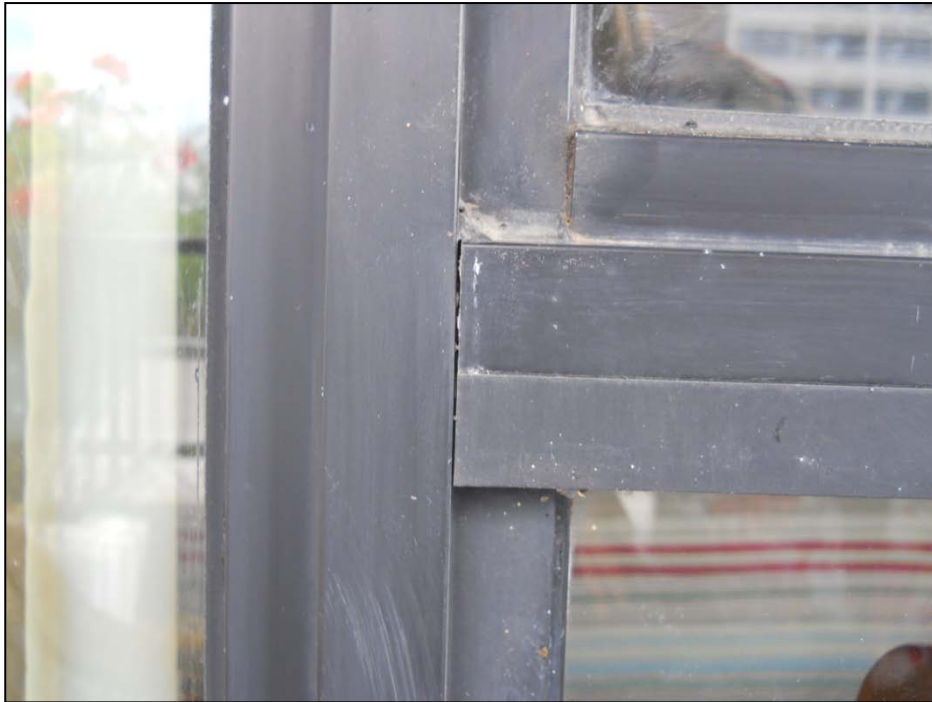
Photograph No. 3: Failed sealed joints within aluminum frame - Suite 407
